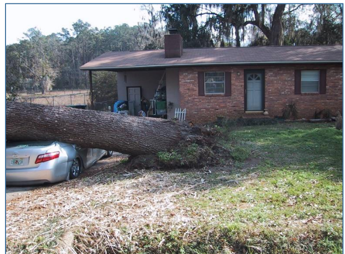
Figure 1. Soil compaction, probably caused by years of parking automobiles under the tree, resulted in root death and tree failure.
