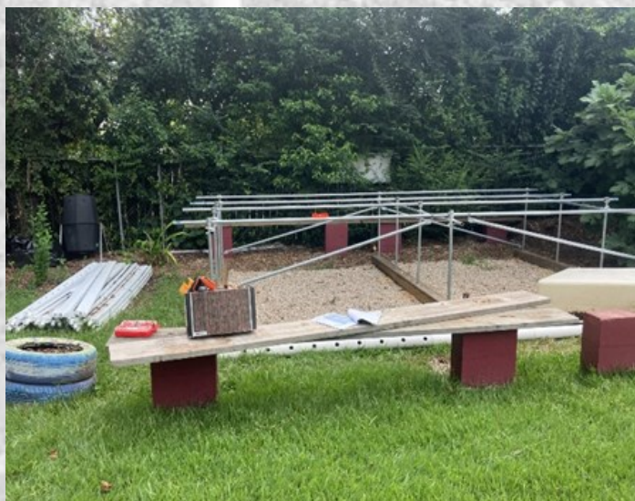
Components of an NFT hydroponic system at the Frenchtown Heritage Hub gardens. From left to right, NFT channels, galvanized steel top rail pipes for the NFT channel support, and other related items.
